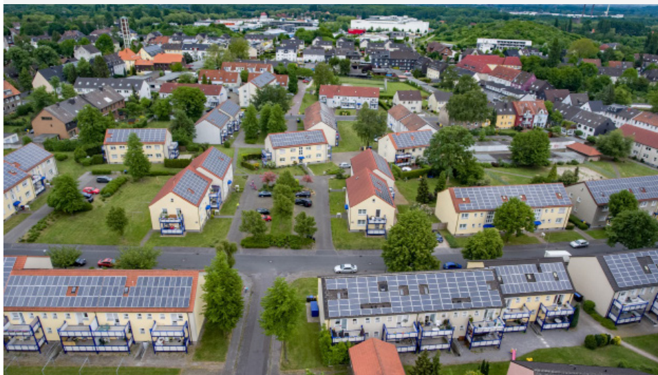
Solarausbau in Bottrop [ICM]
