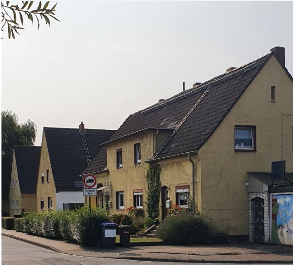
Haus in Fuhlenbrock [ICM]
